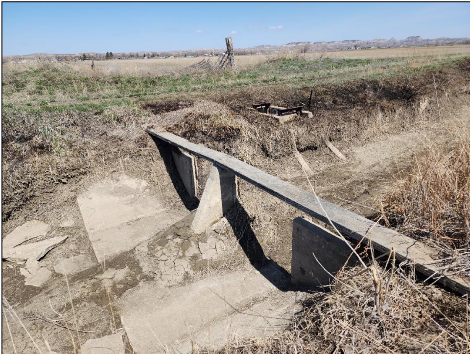
Figure 4: Sluice control, view to the northeast.
