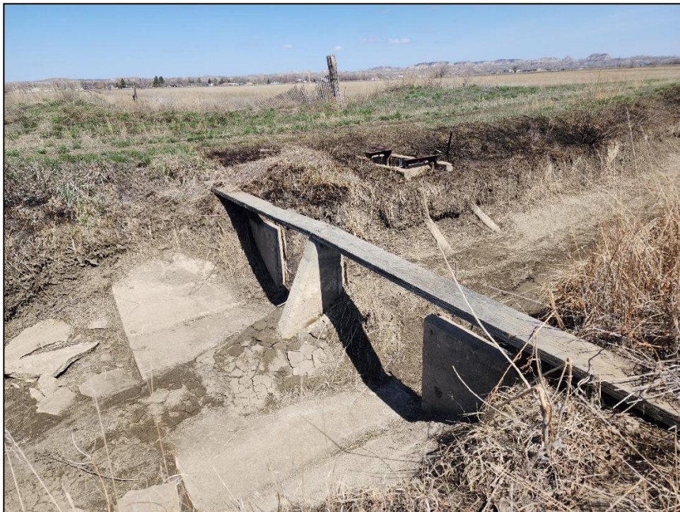
Figure 52: Sluice control, view to the northeast.
