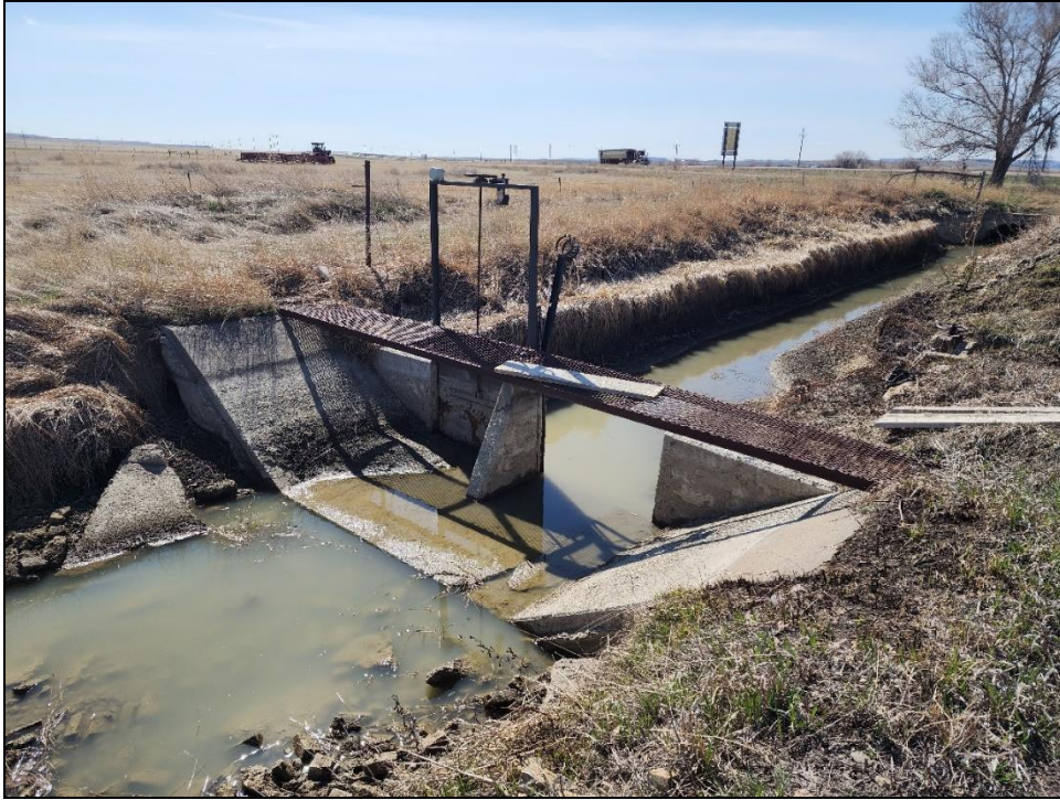
Figure 3: Sluice control near northwest corner of the study area view to the northwest.
